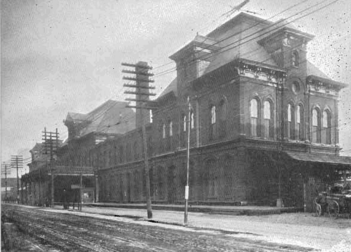
Union Depot—Kansas City, Mo. Erected 1877.
