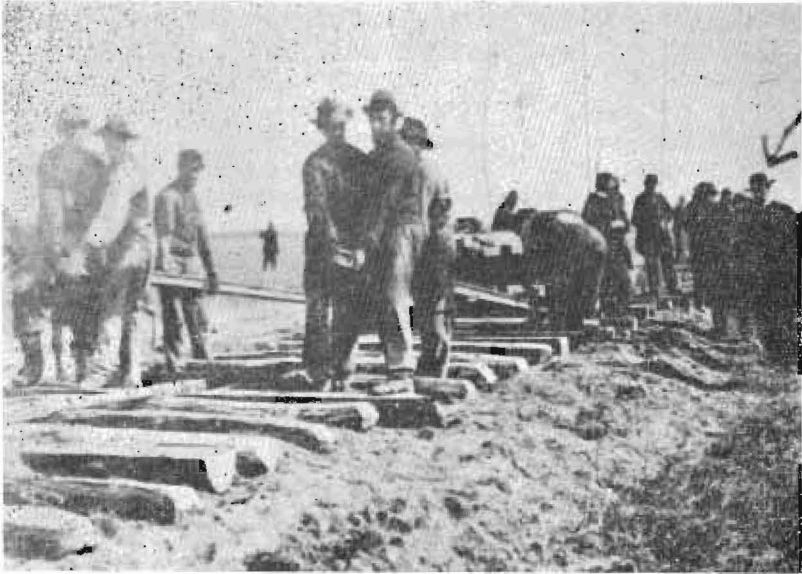
Crew laying track along the Kansas Pacific right-of-way.
