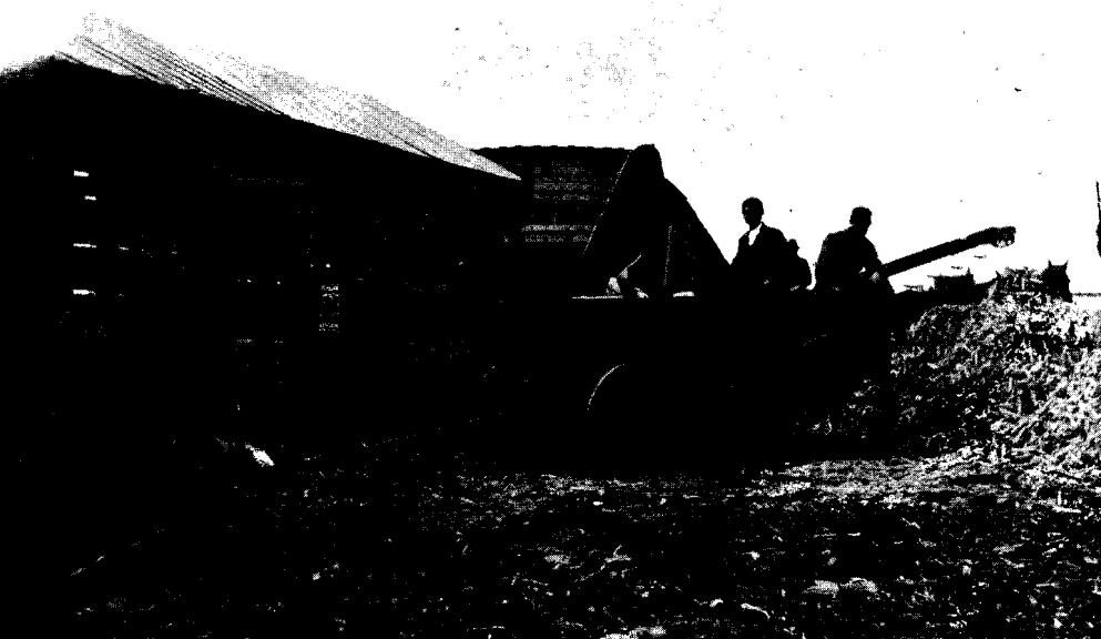
Picture 9: New grain bin built when Cap Ransom started buying and selling grain. (Picture courtesy of Ransom family)
