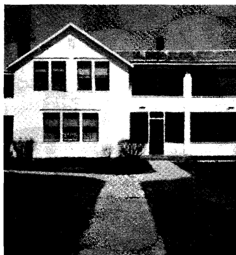
Picture 8: Post Office and General Store as seen today from front.
