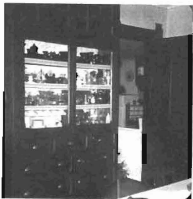
An eight foot tall built-in cabinet in the dining room. Note the small door behind the dishes on the right side. This opens and enables the passing through of food without a trip through the kitchen.
