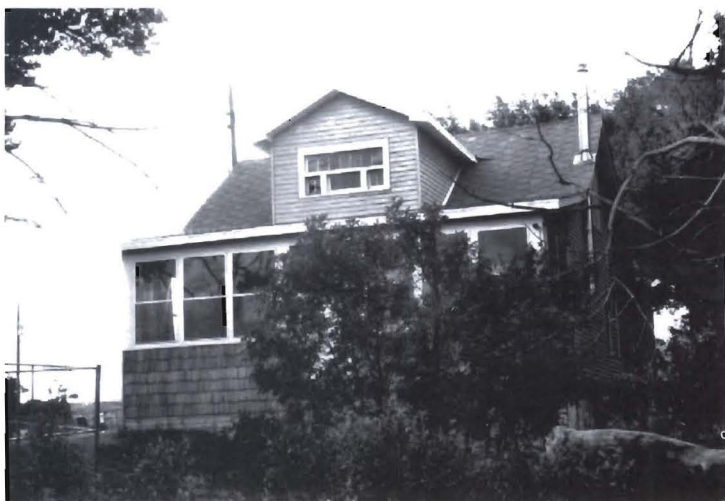
Bradac ranch house on south bank of Little Beaver Creek
