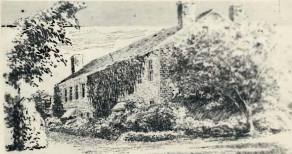
THE HEADQUARTERS OF THE SHAWNEE MISSION INDIAN HISTORICAL SOCIETY. THIS SCHOOL, CHAPEL AND DORMITORY BUILDING OF THE SHAWNEE MISSION GROUP WAS BUILT IN 1832. THE FIRST KANSAS TERRITORIAL LEGISLATURE HELD ITS SESSION IN THE BUILDING IN 1857.
