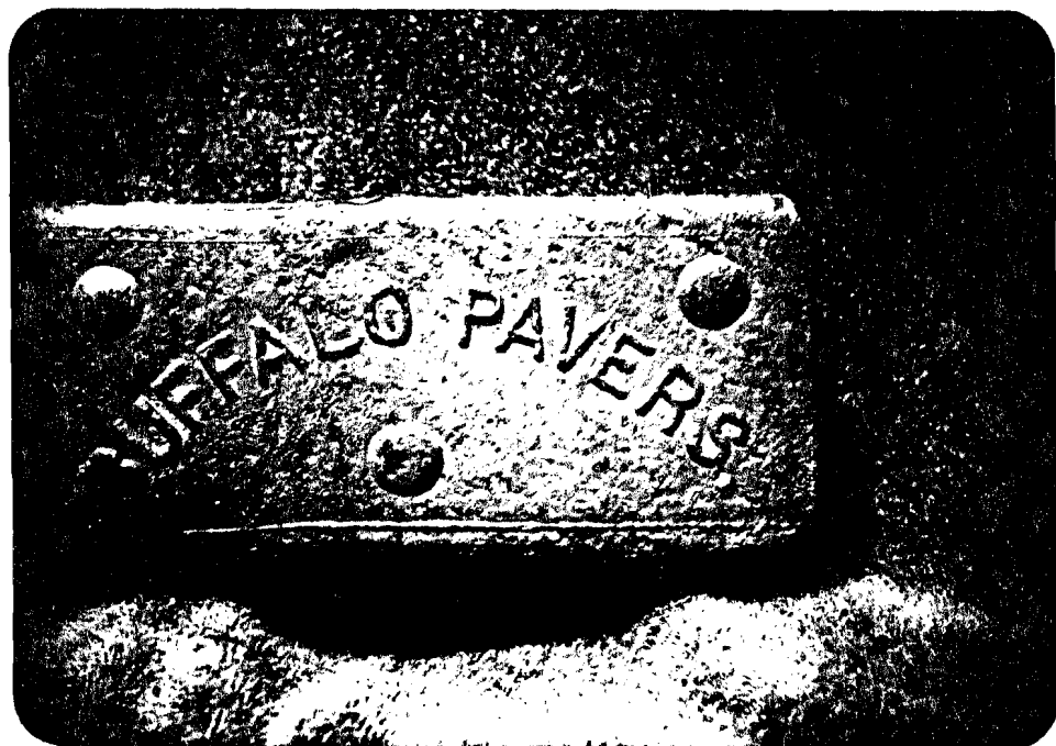
Note the knobs put on some Buffalo street pavers to improve traction.
