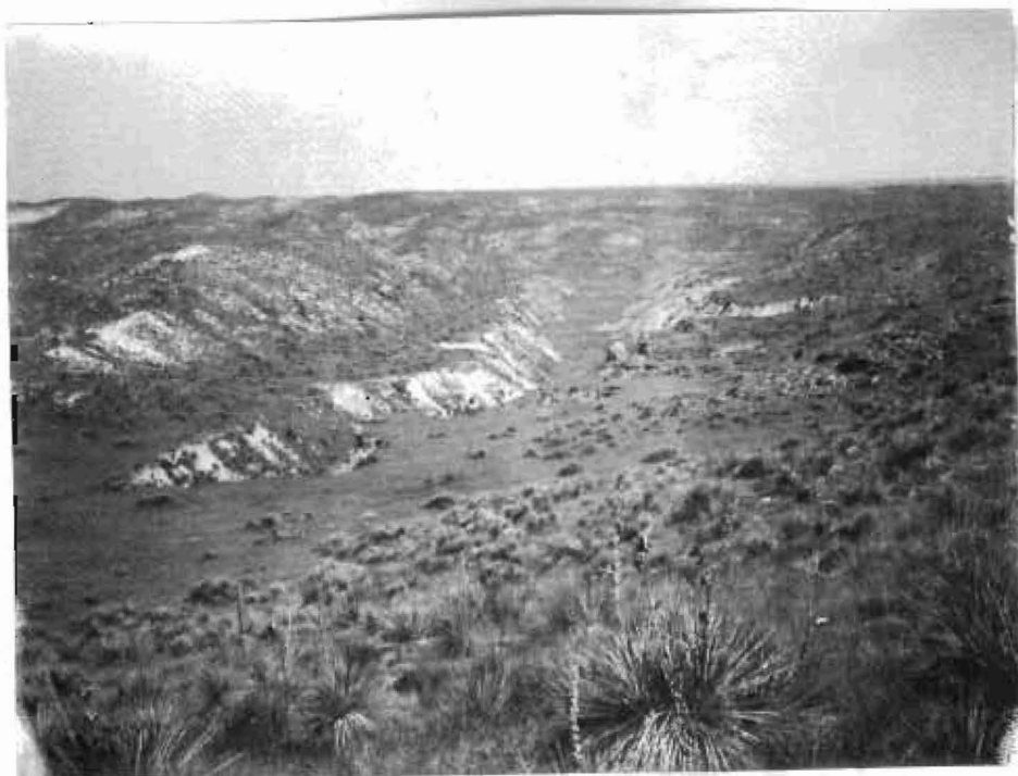
Fig. 4. The crevasse-like drains which extend for miles through the "breaks".
