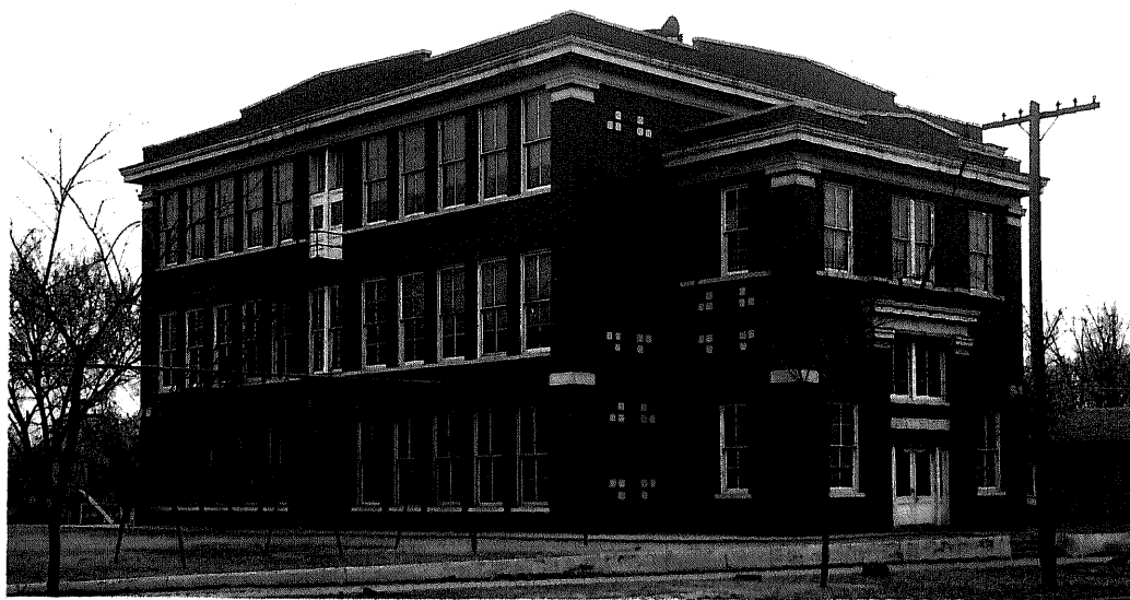
New Lowell Building
