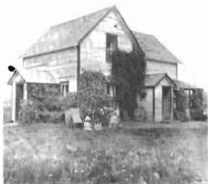
The house at Cottonwood Ranch, ca. 1917
