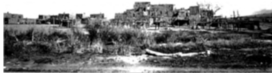
Taos Pueblo, one of the eight Northern Pueblos, is located a mile north of Taos and was the center of the Pueblo community nearly 1,000 years ago. The Taos Pueblo was a multi-storied residential housing, and each home within the adobe structure was self-contained and not connected to other dwellings within the larger building complex. (Wabaunsee County Historical Society)
