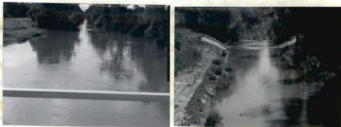
Fig. 8. Station I, Verdigris River, looking downstream towards collection area. During period of normal flow and during period of high-water.
