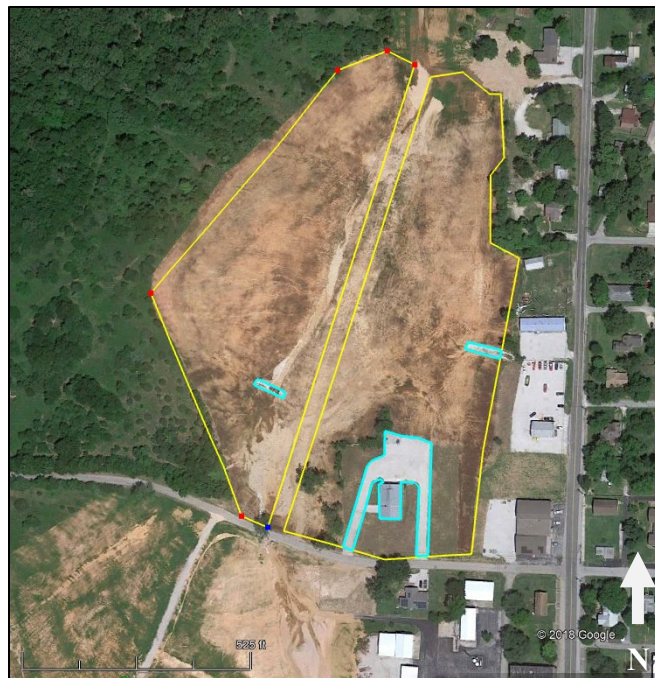
Figure 24. Post-remediation conditions, with total surface area of the west slope as the first subcatchment, referenced as S1-WSlope. (Google Earth, May 24, 2017).
