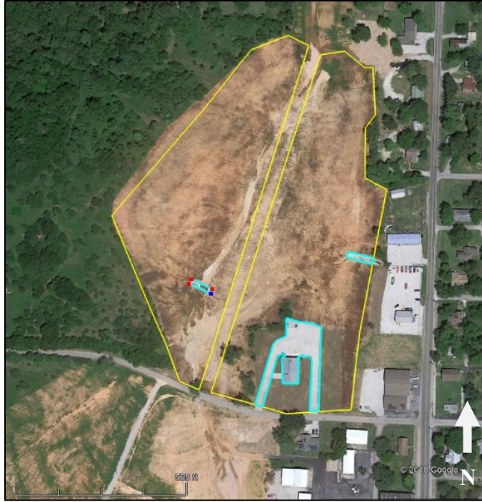
Figure 25. Post-remediation conditions, with surface area of the impervious surface of rock check dam in blue outlines on the west slope. (Google Earth, May 24, 2017).
