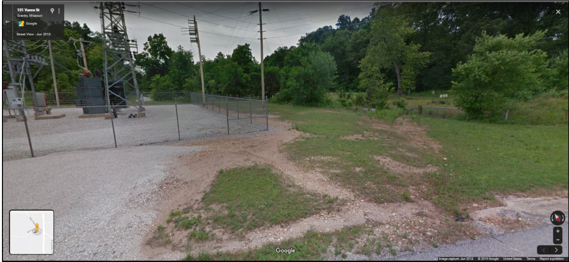
Photograph 3. The northern boundary of the study area as viewed from Vance Street (lower right side and on Figure 2). The pre-remediation tree and grass coverage is visible in this image. The road culvert on Vance Street is also visible in the lower right corner. Facing south, southwest. Photograph is a screen-shot of Google Maps street view dated June 2013.
