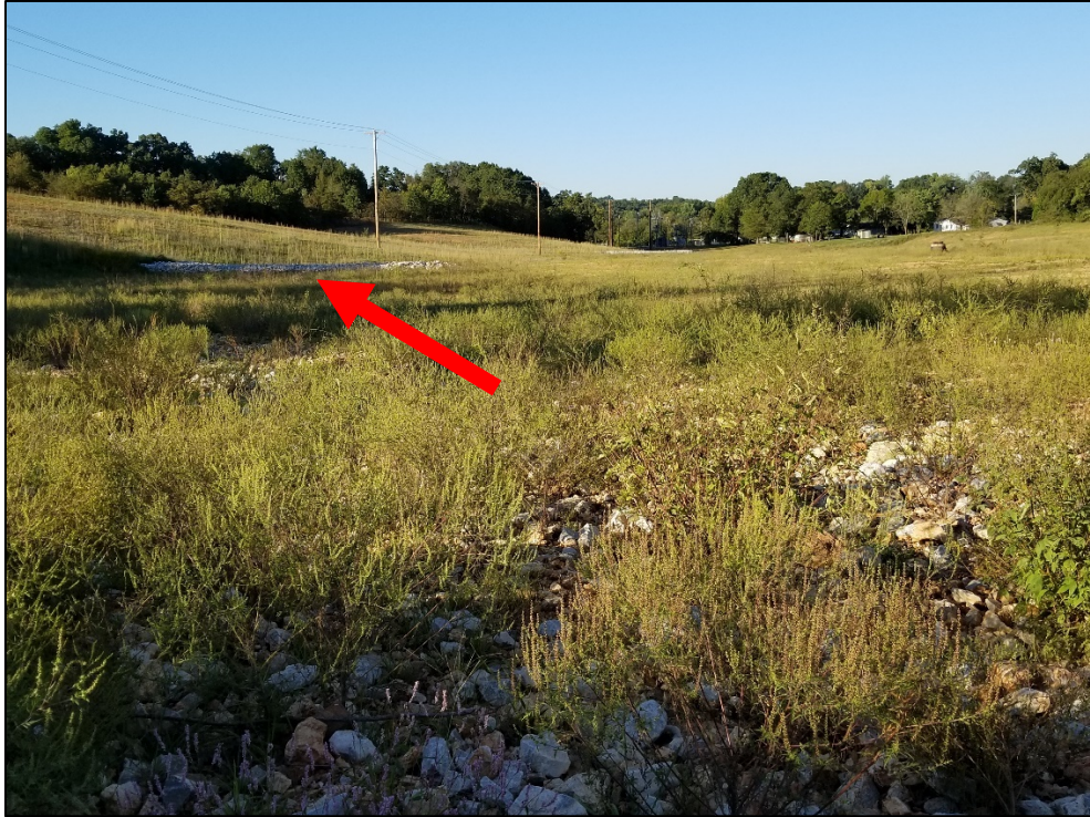
Photograph 4. Rock check dam in top left in the photograph, see the red arrow. Facing north, northwest. (Photograph by Marcia Schulmeister, September 2018).
