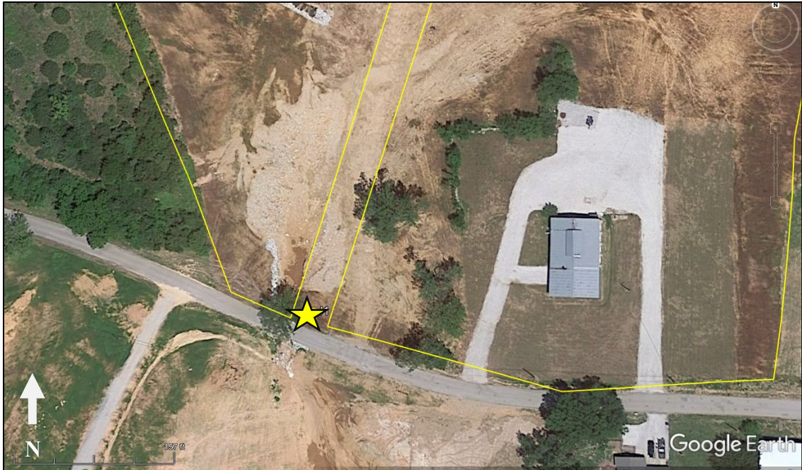
Figure 31. Location of McKinley Street road culvert that is assigned as Junction 1 (J1) in the model. (Google Earth, May 24, 2017).
