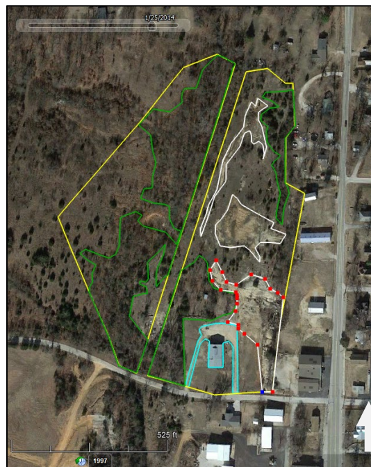
Figure 21. Pre-remediation conditions, with surface area of the southern impervious surface of chat gravel in white outlines on the east slope (Google Earth, January 25, 2014).
