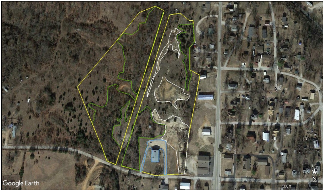
Figure 13. Pre-remediation conditions, with pervious and impervious surface zones defined in this study (colored outlines). (Google Earth, January 25, 2014).
