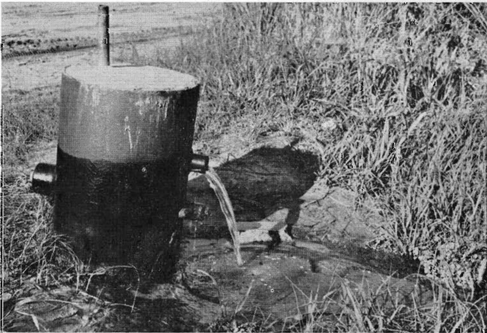
Fig. 3. Artesian well which in part supplied water to boggy marsh.
